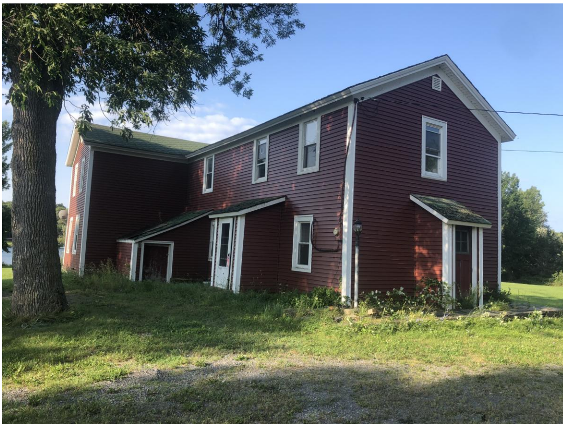
Photograph 4: Northeast oblique of Structure 1 at MDS 1.
