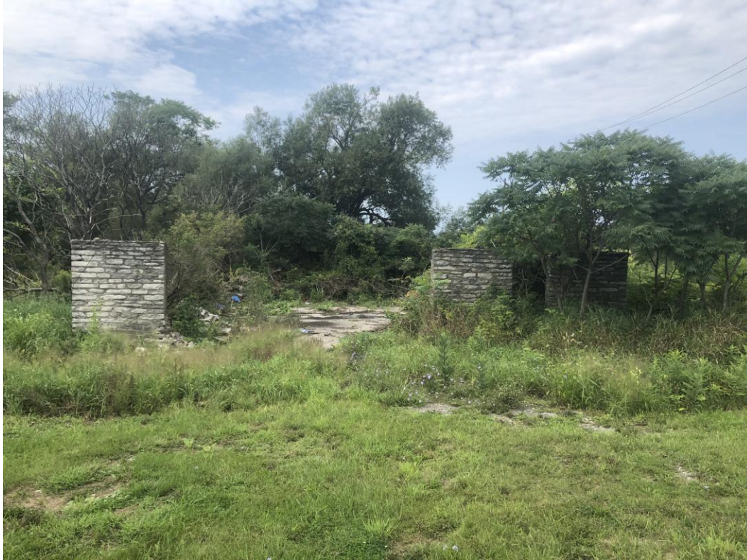
Photograph 5: North face of Structure 2 in at MDS 1.
