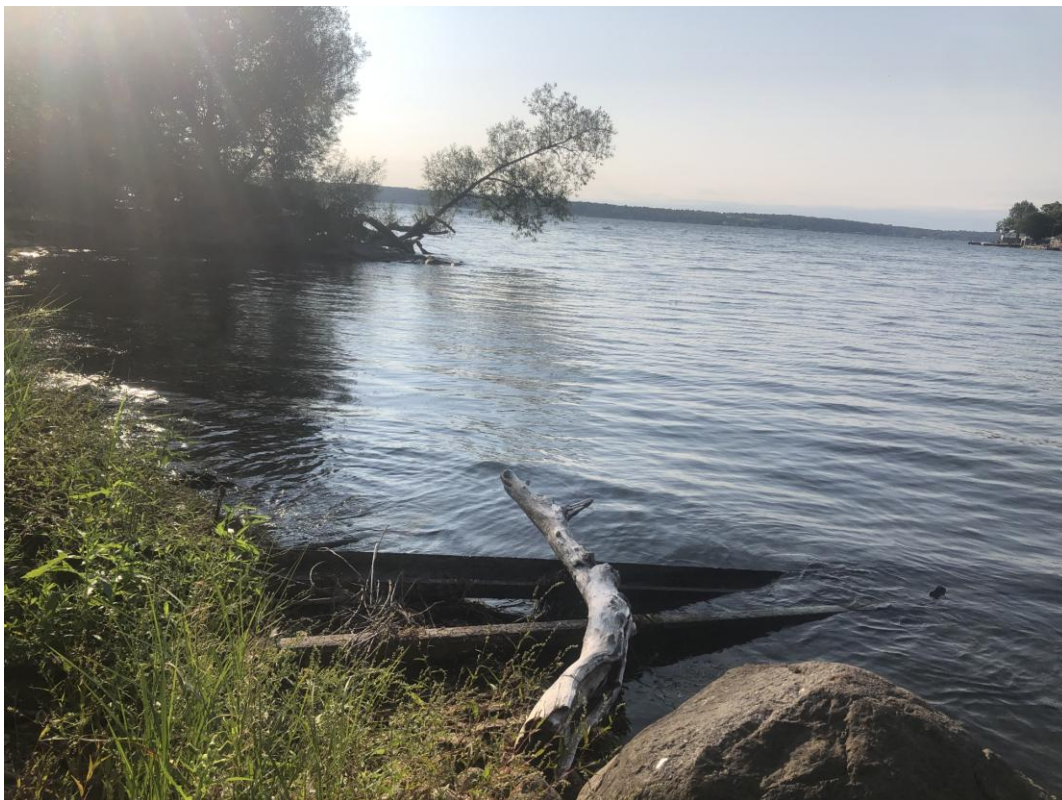
Photograph 8: View southwest of Structure 3 rails and Structure 4 dock and boathouse foundation outside of APE.
