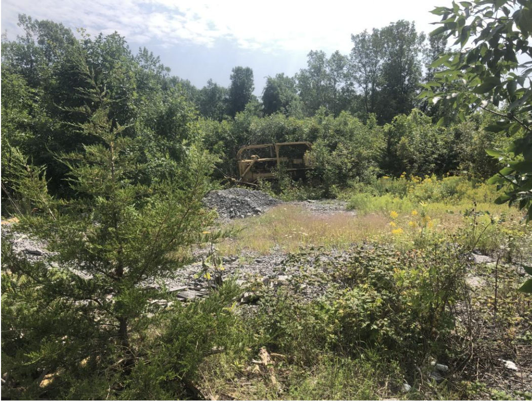
Photograph 13: View southeast of gravel pile and dozer in the central APE.
