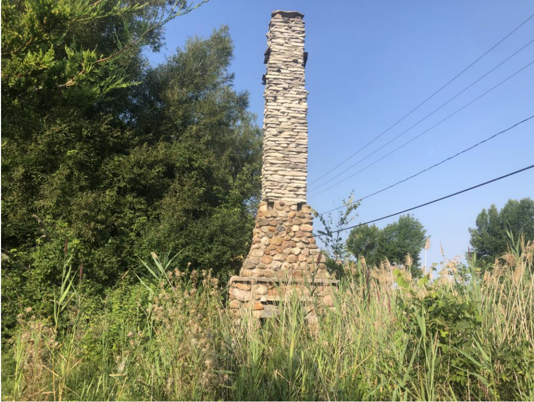
Photograph 9: West view of Structure 6 chimney in northern APE.
